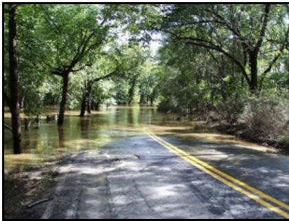
CR 605, Montgomery Twp., Somerset County, after Hurricane Floyd
