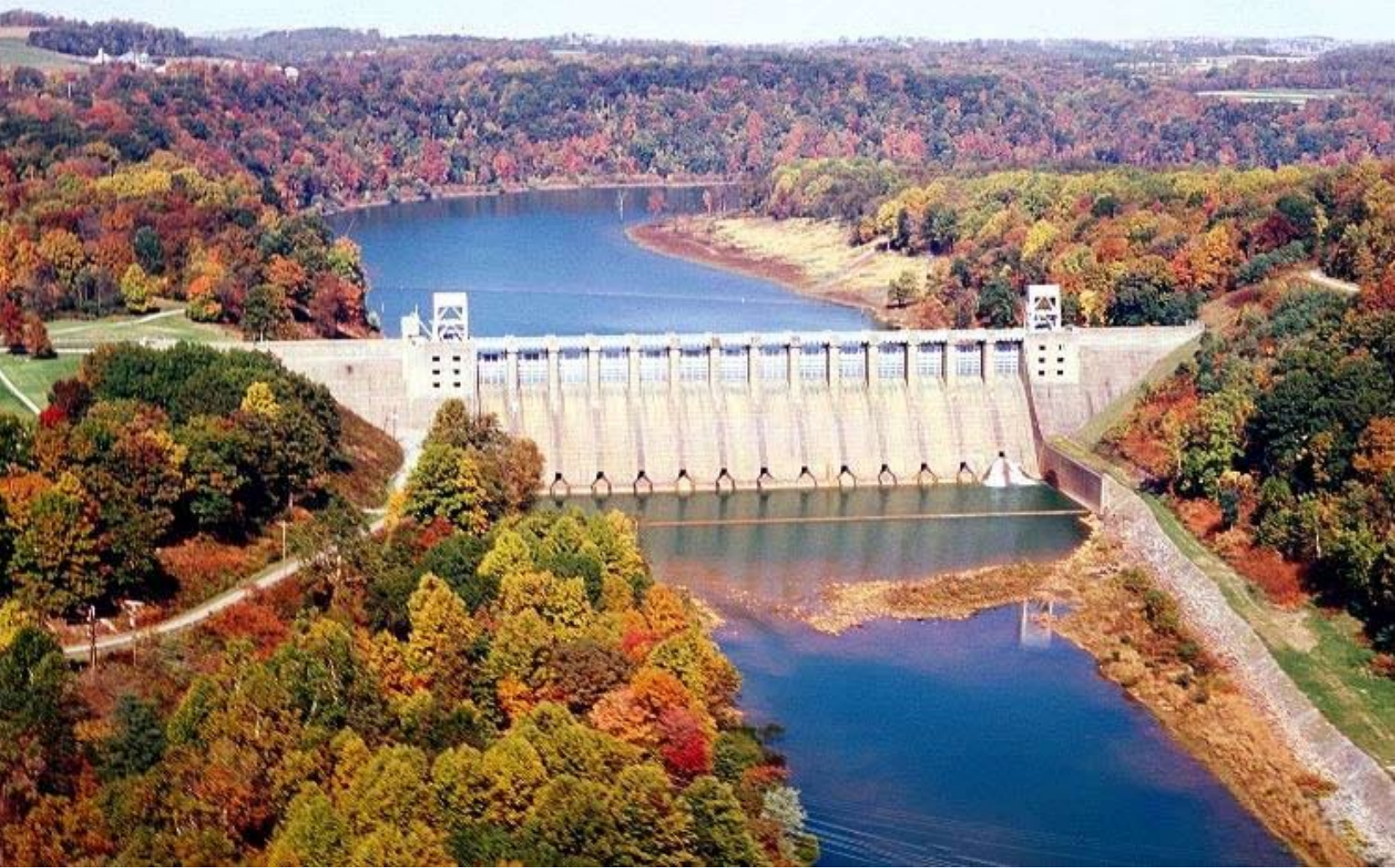
Conemaugh River Lake and Conemaugh Power Plant. Source: U.S. Army Corps of Engineers; Photo by: Margaret Luzier http://corpslakes.usace.army.mil/visitors/projects.cfm?id=H403750 .
